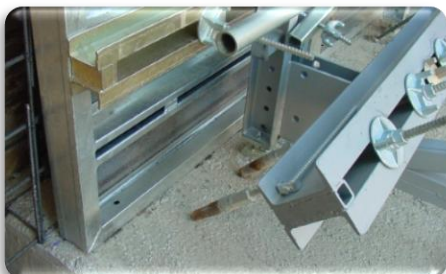
Fixing with dead anchors
