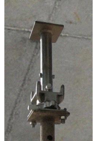
Drop head unlocked on slab
